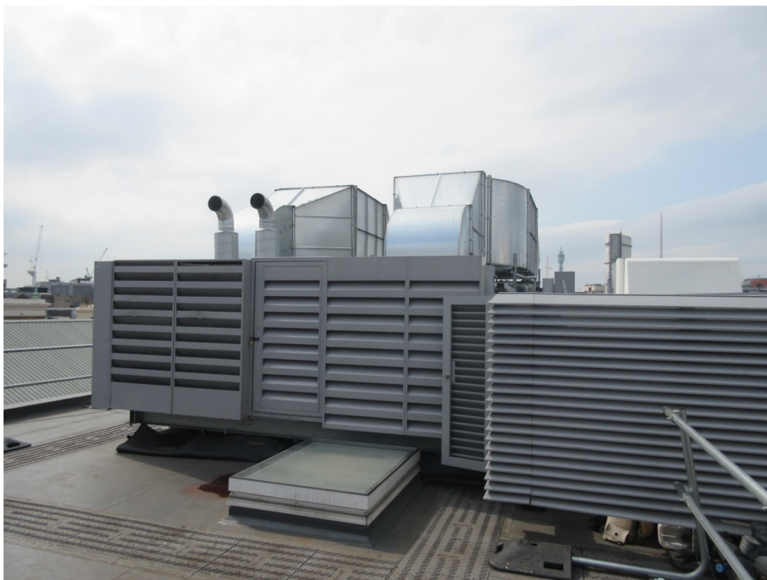
Photo to show rooftop enclosure.
